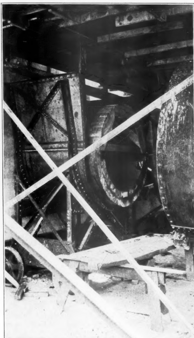
Showing the Cooler Feed End Hood Pushed Back for Lining Lumber Company and the Cross Lumber Company. Pioneer Rubber Mills supplied the belting. Grind-
